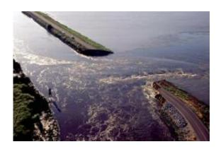
In the summer of 2004, a levee along the Jones Tract in the southeastern Delta collapsed without warning, causing the largely agricultural island to flood. Pumping to drain and restore the island was completed at a cost of more than \$90 million. (Photo courtesy of the California Department of Water Resources)
