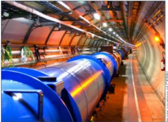
The LHC tunnel
