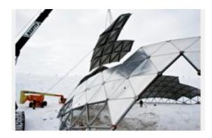
The geodesic dome at Amundsen-Scott South Pole Station was deconstructed during the 2009-2010 austral summer. The materials were shipped to the U.S. Navy at Port Hueneme, Calif., as the dome was built by the U.S. Navy Seebees in the early 1970s. Credit: Forest Banks, National Science Foundation
