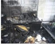
These post-fire photographs of the dorm rooms show the difference a sprinkler makes. There is little visible damage the in the top photo that had a sprinkler in the room; there was no sprinkler in the dorm room in the lower picture. Credit: NIST
