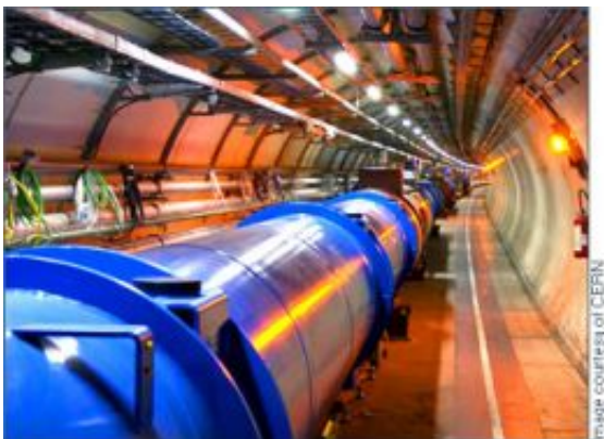
The LHC tunnel
