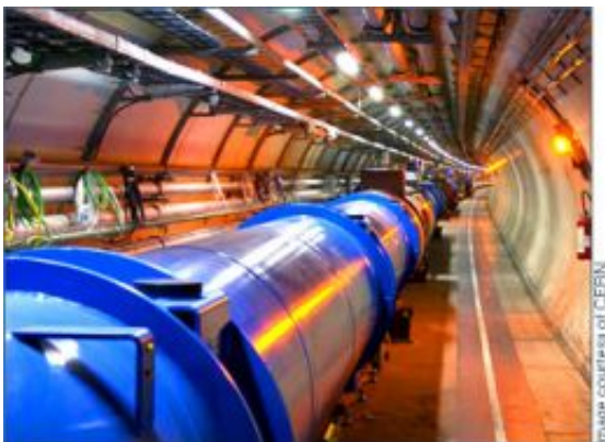
The LHC tunnel
