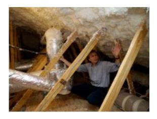
ORNL's Jeff Christian points out the insulating foam used to seal the attic in a deep retrofit house.
