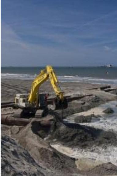
Handout photo shows a bulldozer clearing sand on the beach in Monster in the Netherlands. Sand is being dredged from the bottom of the North Sea off the coast of the country to build dunes as part of an ambitious effort to safeguard the country from flooding.
