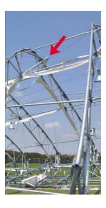
The buckling of the steel frame of the Dallas Cowboys practice facility is seen in the upper left of the photograph (marked by arrow). Credit: NIST
