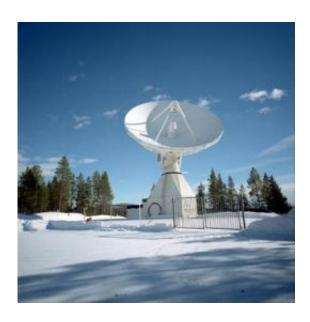
The Kiruna S- and X-band station supports ESA's Envisat and ERS-2 satellites, and is scheduled to support CryoSat-2 in 2009. The station is located at Salmijärvi, 38 km east of Kiruna, in northern Sweden. The station is equipped for tracking, telemetry and command operations as well as for reception, recording, processing and dissemination of data. Credits: ESA - S.Corvaja
