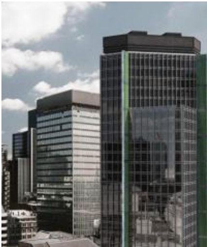
Algae-coated buildings. Image: Institution of Mechanical Engineers
