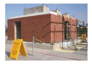
Engineers at UC San Diego will use data from seismic tests of this one-story reinforced concrete masonry structure to help make such structures more earthquake safe. Credit: UC San Diego
