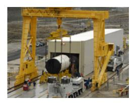
The forward Segment of DM-1 for NASA's Ares I program, is moved into the test stand at ATK facility in Promontory, Utah. Four remaining segments will arrive and be integrated over the next four weeks. Image Credit: ATK
