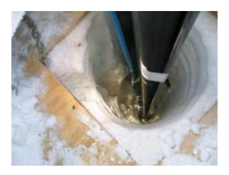
The hot water hose and support cables disappear down one of the dozens of boreholes drilled into the Antarctic ice to construct the IceCube Neutrino Observatory. This enormous telescope is using high-energy neutrinos and cosmic rays to learn about distant cosmological events like supernovas and gamma-ray bursts. Photo: Jim Haugen
