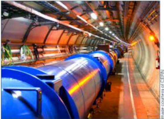
The LHC tunnel
