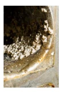
Struvite, a phosphate mineral, clings to the interior walls of a heat exchanger at the Madison sewage treatment plant. Photo: Bryce Richter
