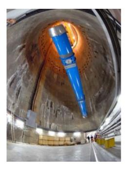
The last of 1746 superconducting magnets is lowered into the LHC tunnel via a specially constructed pit at 12:00 on 26 April. This 15-m long dipole magnet is one of 1232 dipoles positioned around the 27-km circumference of the collider. Dipole magnets produce a magnetic field that bends the particle beams around the circular accelerator. Photo / CERN
