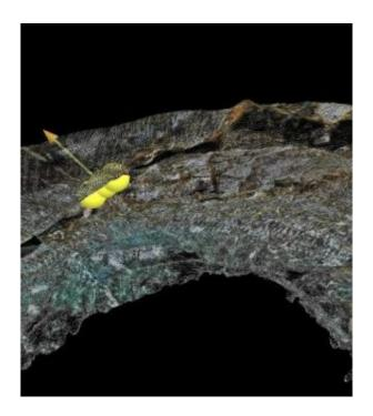
Close-up image of the tunnel roof showing a gVT measurement location. The arrow is a vector perpendicular to a surface that marks a discontinuity between rock layers. The orientation of the arrow in space gives the azimuth and slope of the surface. Credit: Jeramy Decker, Kiewit Corp
