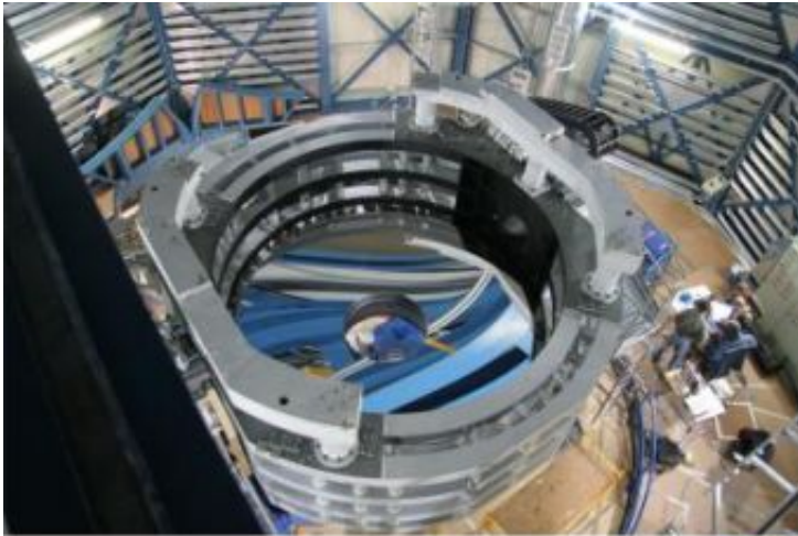
The VISTA Mirror Installed
