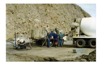
Preparing to cement an experimental geophone string in a borehole in Central Queensland. Image credit – CSIRO
