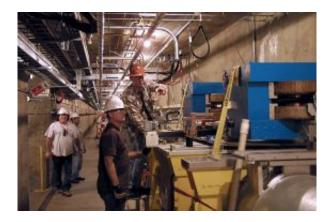
Crews working in the linac tunnel install two 4,000-pound magnets as part of the second bunch compressor for the LCLS.
