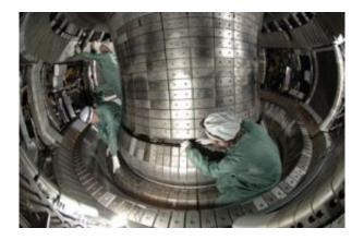
Tungsten-clad wall tiles being installed in the plasma vessel of ASDEX Upgrade (Photo: IPP)
