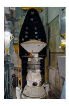
On Launch Pad 17-A at Cape Canaveral Air Force Station in Florida, the first half of the fairing is installed around the Phoenix spacecraft. NASA/George Shelton
