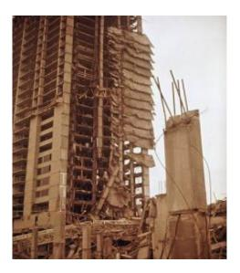
The Skyline Plaza Apartments in Fairfax County, Va after a 1973 progressive collapse that occured during construction of the 24th floor. The collapse involved the full height of the tower, and falling debris also caused the horizontal progressive collapse of an entire parking garage under construction adjacent to the tower. Fourteen workers were killed, 34 workers were injured. Credit: Hai S. Lew/NIST
