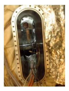
Shyri Marazita, an engineer at the MIT Plasma Science and Fusion Center, peers out of the Alcator C-Mod vacuum vessel. He is in the process of installing a liquid helium cooled cryopump, a modification that will help the reactor achieve a steady-state flow of plasma. Photo: Donna Coveney
