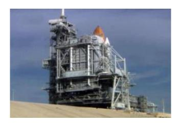
The rotating service structure is in place around Space Shuttle Discovery at Launch Pad 39B, leaving only the top of the external tank and boosters visible. Image Credit: NASA
