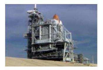
The rotating service structure is in place around Space Shuttle Discovery at Launch Pad 39B, leaving only the top of the external tank and boosters visible. Image Credit: NASA
