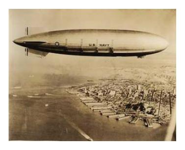
Like its sister ship, the USS Akron (shown here flying over the city of San Francisco), the USS Macon was a familiar sight across the United States. Thousands of people would turn out to observe the "flying aircraft carrier" conducting training maneuvers. The USS Macon was constructed with a built-in aircraft hangar and a trapeze launch and recovery system to facilitate fighter planes intended to protect the aircraft in war. Image credit: Wiley Collection, Monterey Maritime and History Museum
