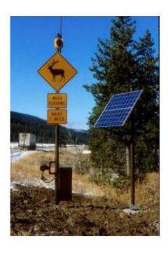
As part of a six-year study, the Western Transportation Institute at Montana State University helped test and develop this animal-detection system on U.S. Highway 191 in Yellowstone National Park. The system reliably detects elk on, or near, the roadway ahead and warns drivers. Credit: Photo by Marcel Huijser, WTI-MSU
