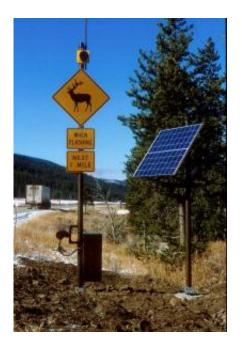
As part of a six-year study, the Western Transportation Institute at Montana State University helped test and develop this animal-detection system on U.S. Highway 191 in Yellowstone National Park. The system reliably detects elk on, or near, the roadway ahead and warns drivers. Credit: Photo by Marcel Huijser, WTI-MSU
