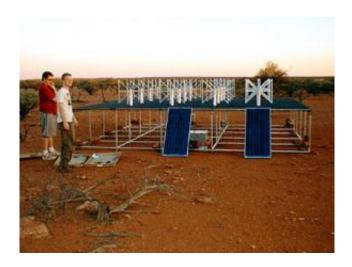
Students help construct a prototype in April 2005 of one of the 500 'tiles' that will make up a new telescope in Australia. Each tile consists of 16 antennas. From left are Jamie Stevens, a graduate student at the University of Melbourne, now at University of Tasmania, and Judd Bowman, a graduate student in physics at MIT. Photo / Merv Lynch, Curtin University of Technology, Australia
