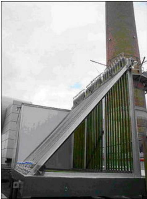
Figure 1: Early prototype bioreactor on the roof of the MIT cogeneration plant. Greenfuel has advanced the design and scale since. Cambridge, Mass (photo courtesy of: the http://fraserdomain.com )
