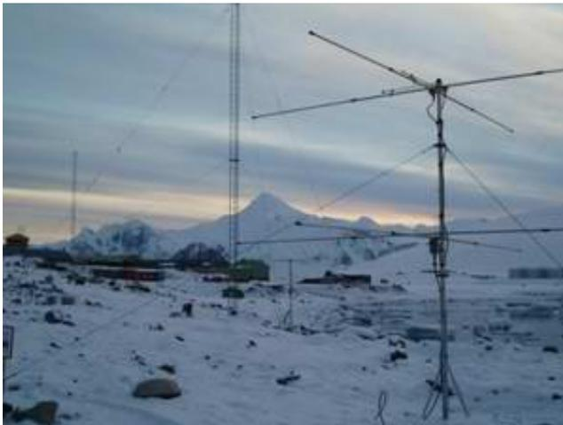
A new research radar based in Antarctica is giving scientists the chance to study the highest layer of the earth's atmosphere at the very edge of space.
